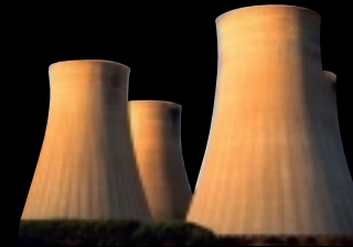
Brazing of copper parts in generators. Shrink- fitting. Bolt expansion. Pre/post heating and brazing for high-pressure turbines.
